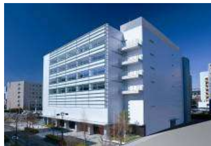
R&D Center and Head Quarters at Shin-yokohama
