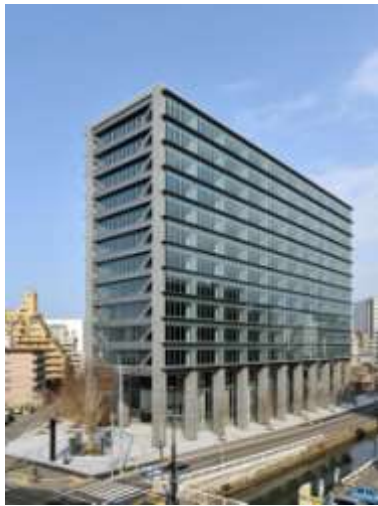
▲ External appearance at Fukuoka Lab.
